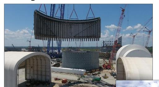
Placement of the In-containment refueling water storage module, VC Summer Unit 2
